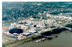
Bulk Fuel Storage
